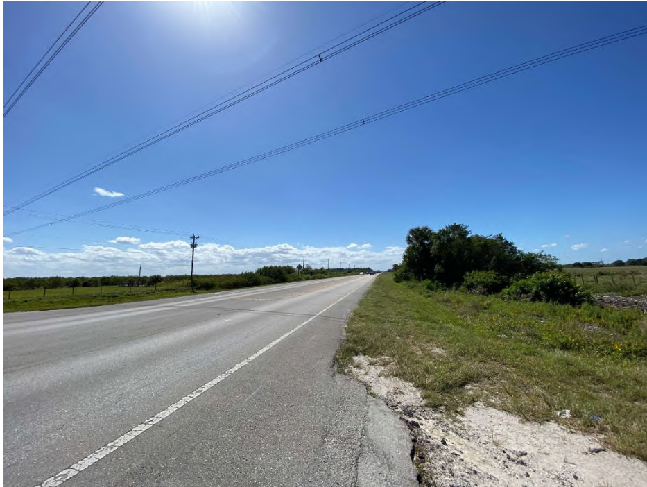
Survey Station No. 2 – View to South
