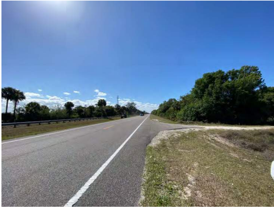
Survey Station No. 10 – View to South
