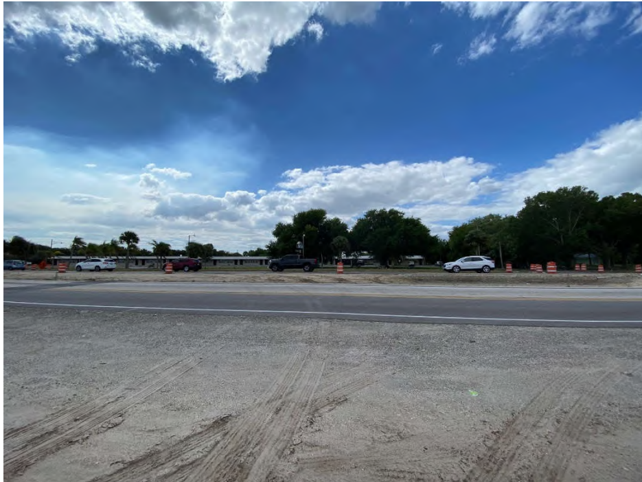
Survey Station No. 1 – View to South
