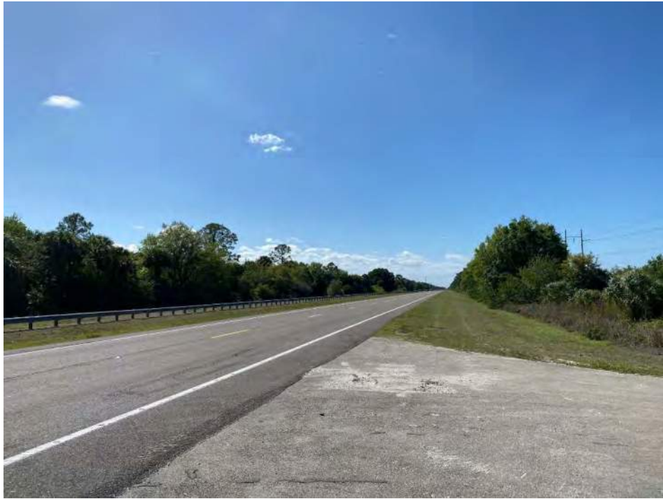
Survey Station No. 8 – View to South
