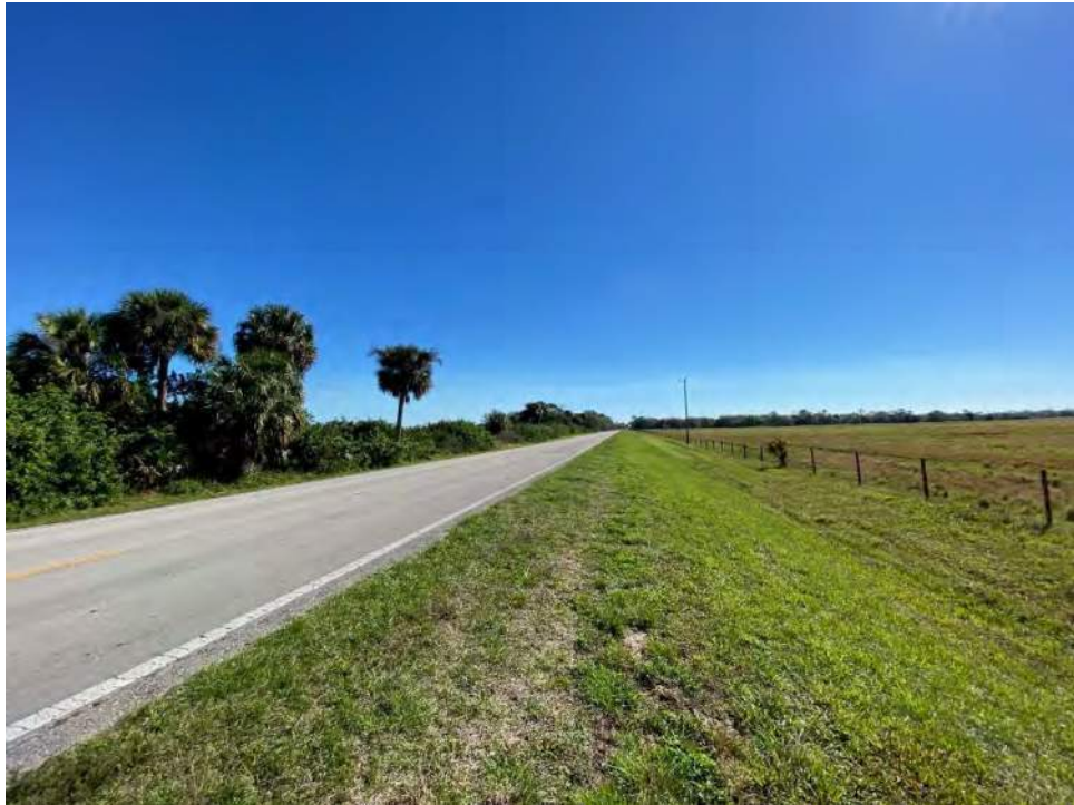
Survey Station No. 12 – View to South
